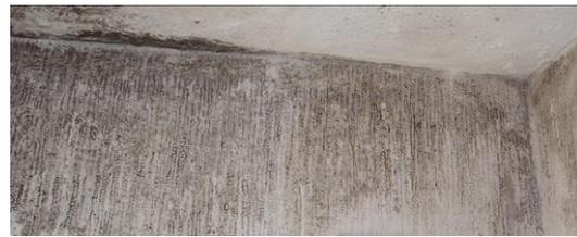
Unsurprisingly, black spot mould growth can usually be found around windows where the external skin of masonry is in touch with the internal skin of a cavity wall forming a cold bridge, in the corners of rooms, behind or even within cupboards and wardrobes where air doesn't circulate well.
