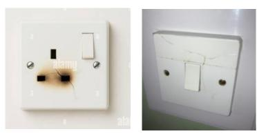
Any switches, socket outlets or pendant which have cracks or sections missing will need to be replaced.
